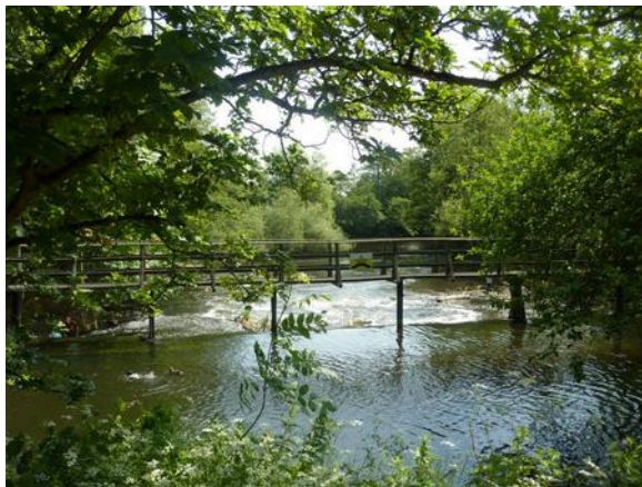
The wooden footbridge by the weir at Darley Abbey
