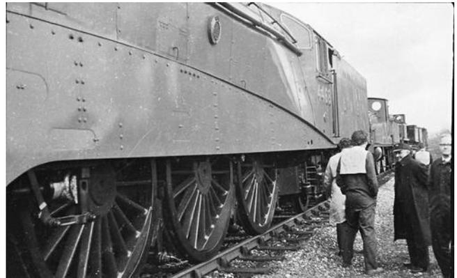
The first inspection stop. Why is Mallard getting all the adulation whilst I am slogging up and down the train checking axleboxes, suspension and brakes?
